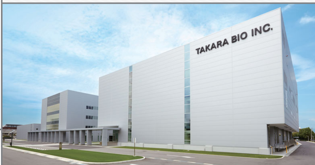
Consolidating research sites into a new facility
